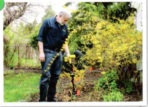
The exact location and depth of the pipe run and its fittings is also determined with the use of specialized locating equipment that reads a signal transmitted by the camera when it is inside the pipe.
