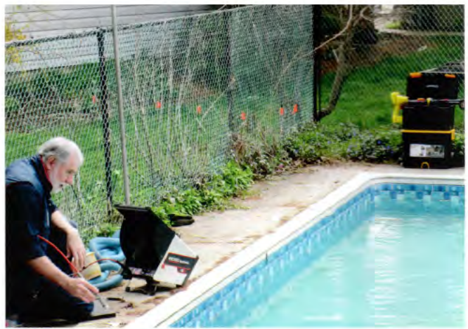
The camera inspection also helps to locate the route of the plumbing lines.
