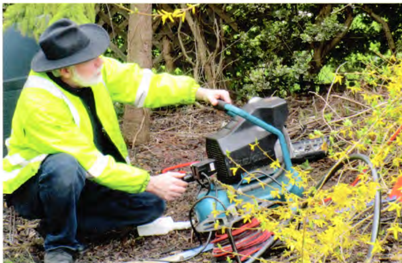
Pressurizing a suspect line involves plugging the jets/skimmer and disconnecting the pipes near the pump to apply a combination of compressed air and water while monitoring the gauge for results.
