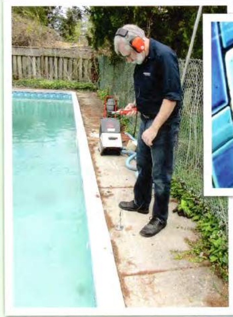
After pressurizing the lines, sophisticated microphones are used to listen above ground and underwater for the sound of escaping water and air.
