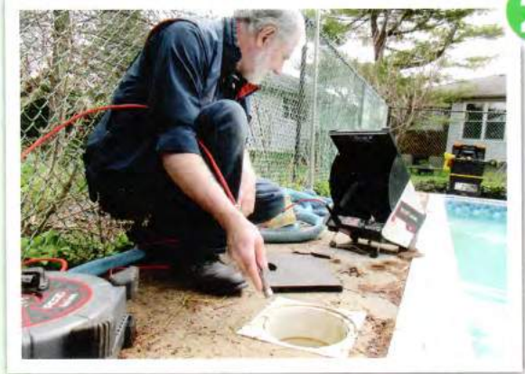
The exact location and depth of the pipe run and its fittings is also determined with the use of specialized locating equipment that reads a signal transmitted by the camera when it is inside the pipe.
