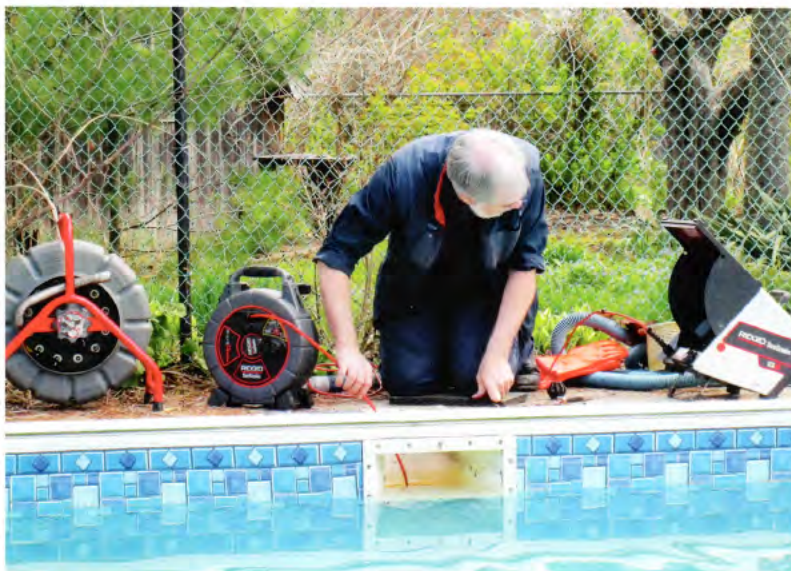
A camera is used to inspect the skimmer line.
